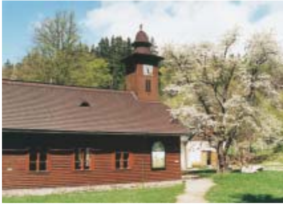
THE BUILDING IN WHICH THE MINERS GATHERED PRIOR TO THEIR SHIFT, PART OF THE SURFACE EXHIBITION OF THE OPEN AIR MINING MUSEUM (SKANZEN)
