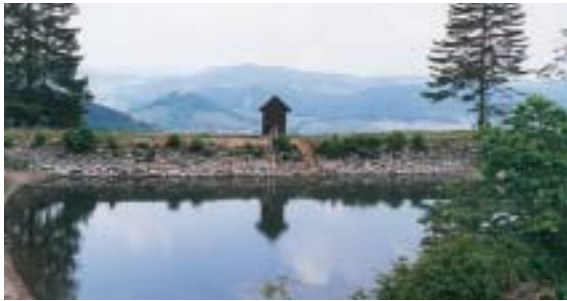
THE OTTERGRUND RESERVOIR ON THE SLOPES OF PARADAJZ HILL IS ONE OF THE SMALLEST AND ALSO THE HIGHEST OF THE RESERVOIRS AND ITS DAM GIVES SPLENDID VIEWS OF THE TOWN (SEE ALSO THE SECTION – 7 BANSKÁ ŠTIAVNICA WALKS)
